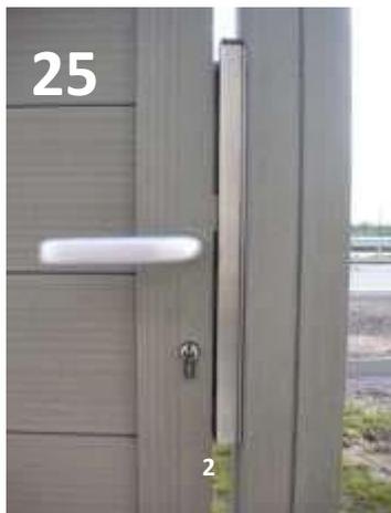
**25** When the gate hangs into the hinges and the gate is closed, the latch bolt should be in the middle of the latch bolt opening.
