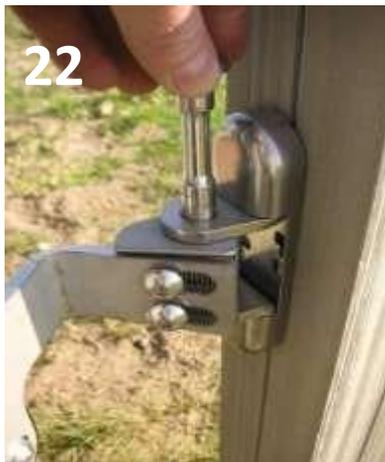
**22.** Place the gate in the hinges and slide the pin down into the hole.
