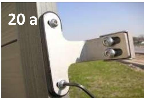
**20a** Attach the hinge to the gate.
